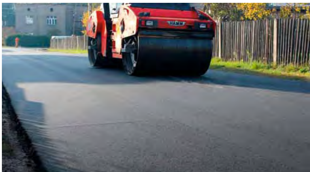
Figure 6.7. Placement of experimental section with ORBITON 65/105-80 HiMA in 2013.
